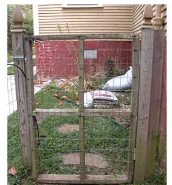
Wood gate with welded wire stapled to it
